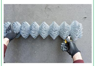
**Step 1:** Cut the tying wires that are used to fasten the roll and keep it from unraveling. Do this carefully so that you don't cut into the mesh itself.
